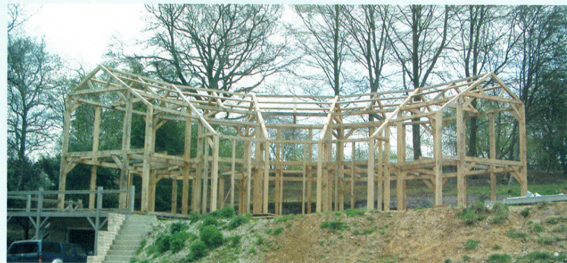
The completed frame has echoes of the reconstructed Globe Theatre
