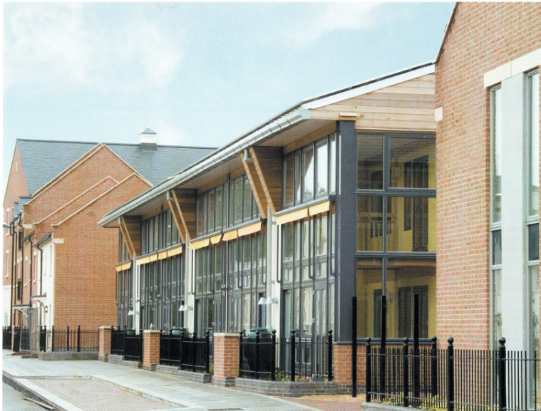
The first housing development built to meet Code Level 6 using the ruralZED™ zero carbon housing system is in Northampton.
