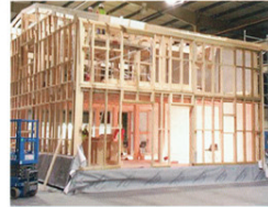
External studwork modules and membrane installation.
