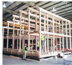
Assembled glulam frame.
